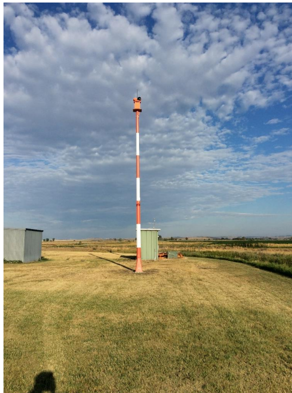
Airport Rotating Beacon
